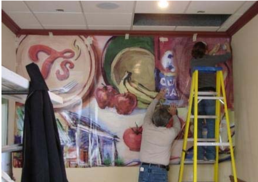
Scott from Graphic Innovations installing the “Mural” in EG
